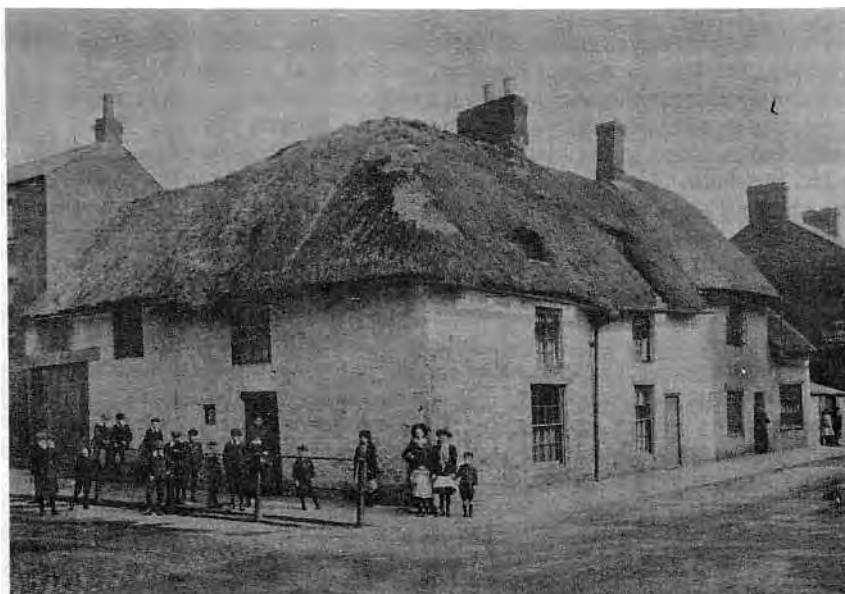
The corner of Broad Street and George Street showing the entrance to Church Court
