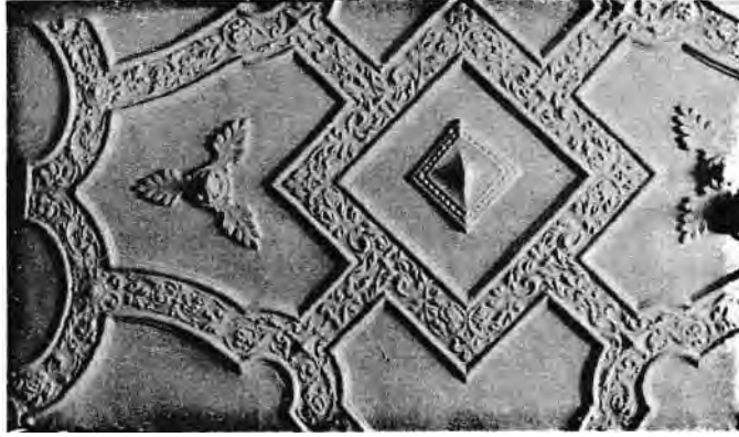
The ceiling at the Britannic Assurance Company's office on the Green, Banbury (photograph: Gretsel Press)
