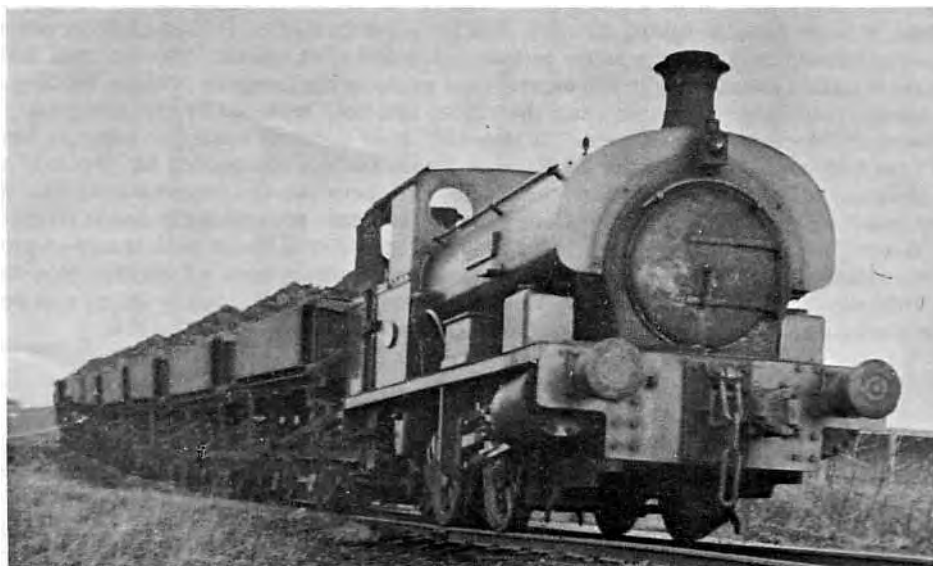
Figure 3. 0-4-0 Locomotive "Barabel" approaches the crushing plant from the quarries. 1955. (B.S. Trinder).
