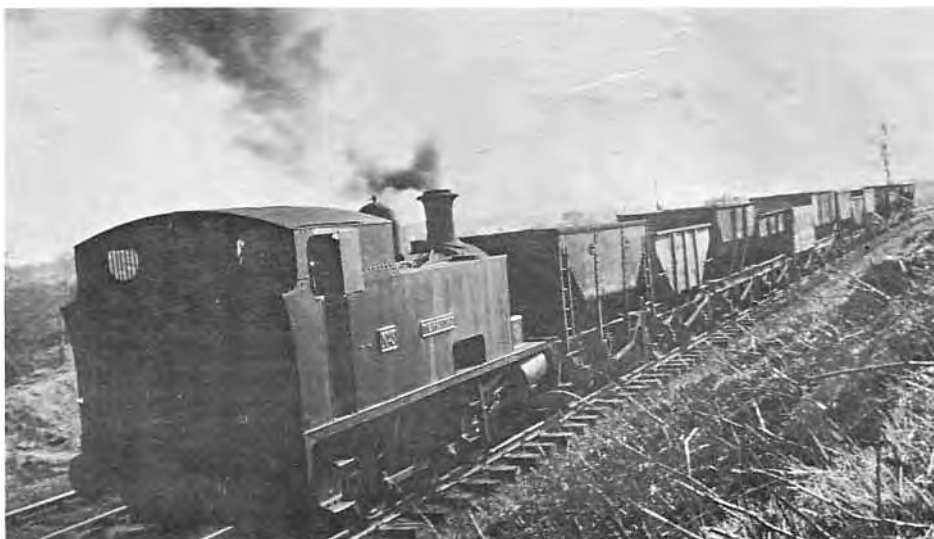
Figure 4. 0-6-0 Locomotive No. 3 "The President" pushes empty British Railways hopper waggons up the "main line" towards the Wroxton crushing plant. 1955. (B.S. Trinder).
