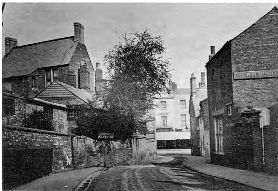
Fig. 7. Marlborough Road looking into the High Street, in April 1910. Note the laburnum tree. (B.20)
