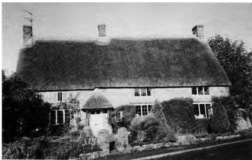
Cottage in Cropredy (30th September 1993). Grade II listed building. Historic Building grant made for thatching.
