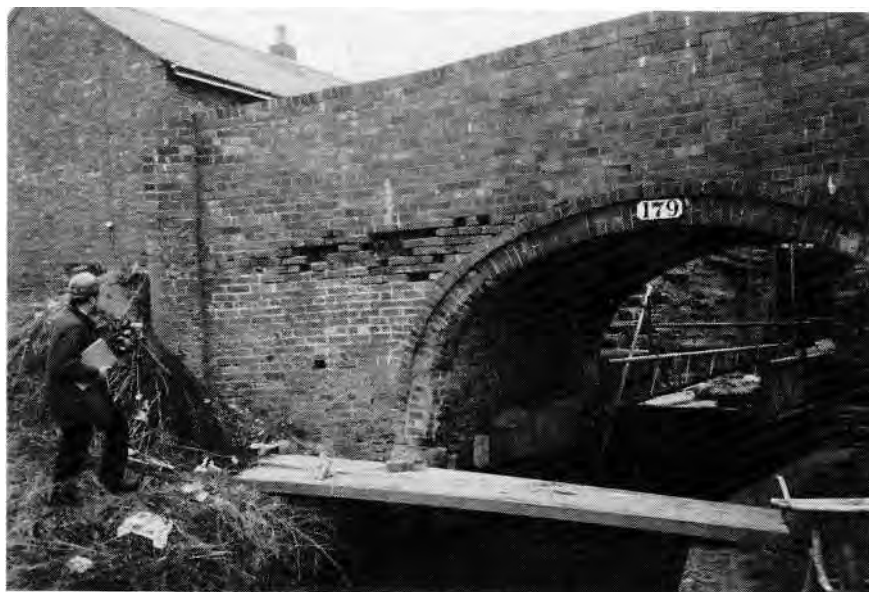
British Waterways: Repairs to Kings Sutton Lock and Bridge (12th February 1993); Grade II listed canal structure.
