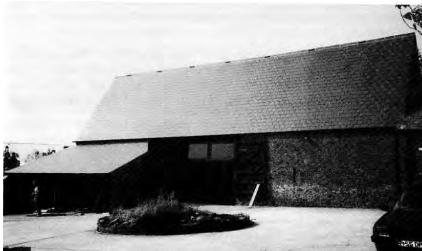
Barn at Wykham Mill Farm, Banbury (13th September 1991). Sympathetic conversion to showroom for Jaguar Sport.
