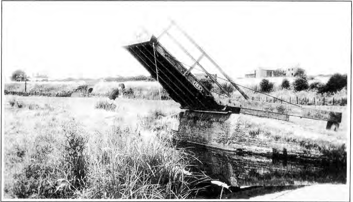
Oxford Canal near Adderbury, looking south. To the left of the picture, just out of sight, is the site of Railton's wharf. In the middle is the formation (embankment) of the Banbury to Cheltenham railway and in the distance is Sydenham farm.
