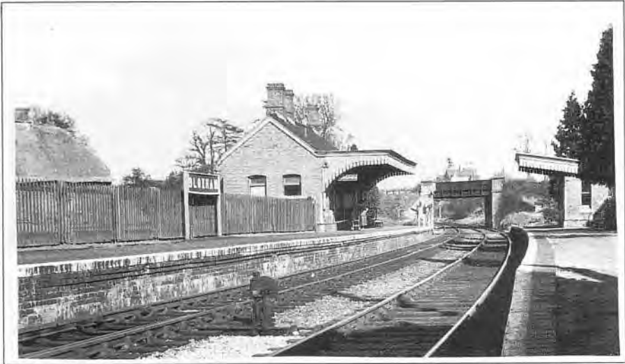
Bloxham station, located at the south-western limit of the village, looking east towards Adderbury. The Banbury and Chipping Norton road crossed the railway on the girder overbridge beyond the platform, the fourth bridge to cross the line from Adderbury within a short distance. The single line staff set down and pick-up posts (and the lamp post) can be seen at the far end of the up platform, in front of the bridge L & GRP
