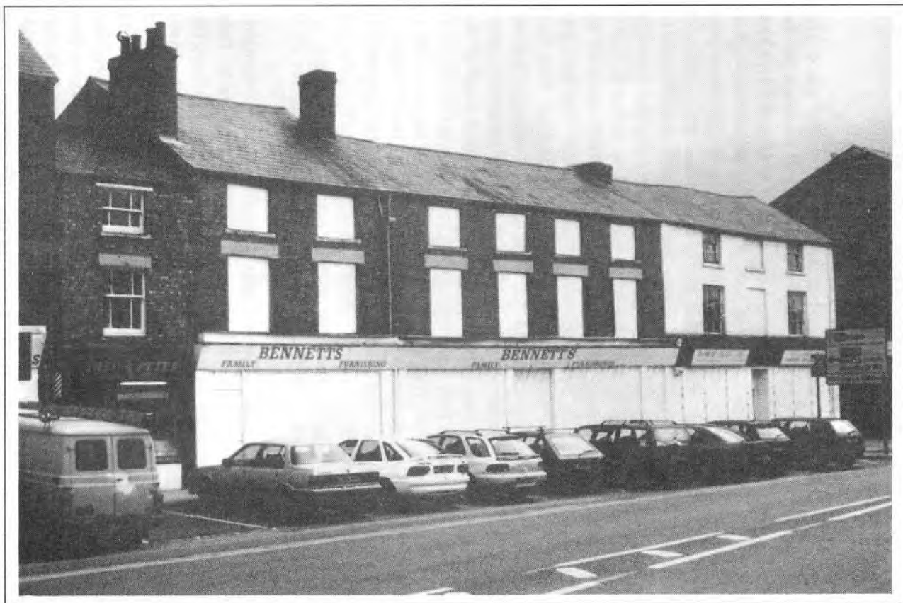
Plate 5. The facades of 53 and 54 Bridge Street.
