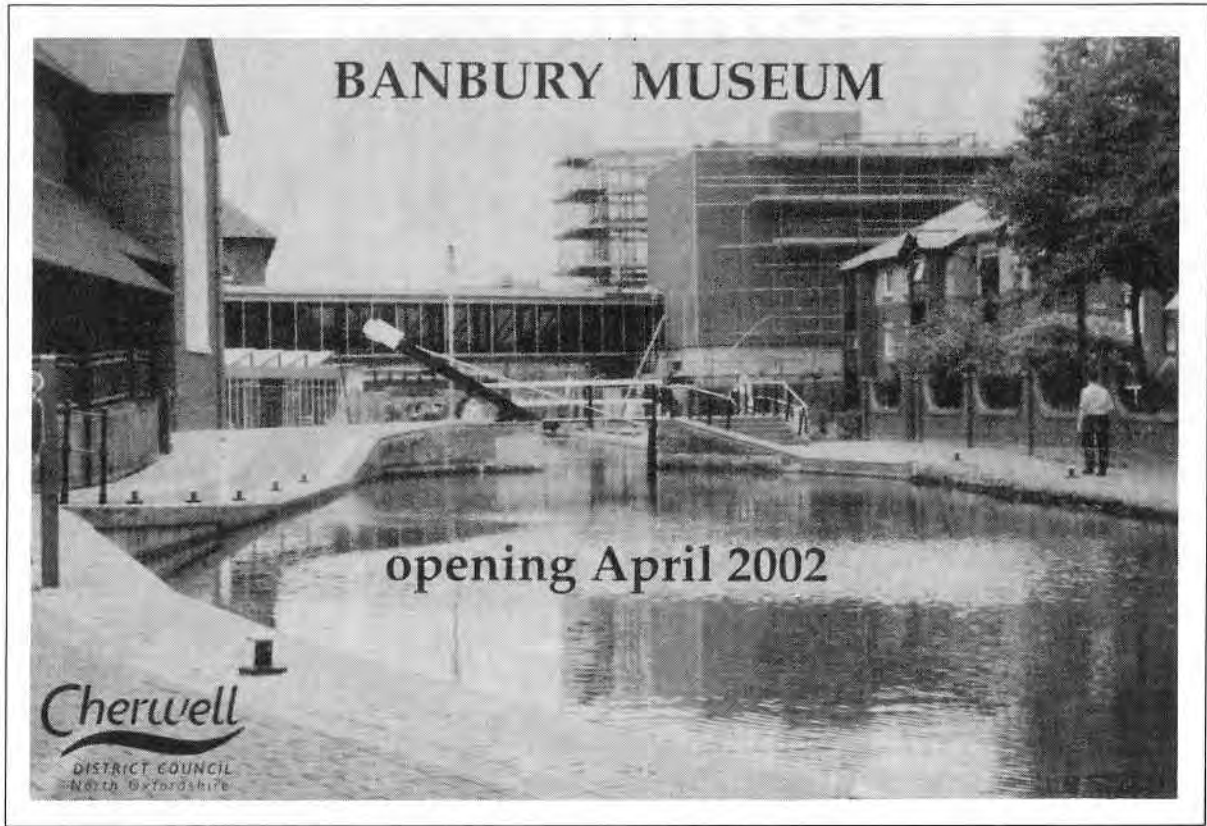
The new Banbury Museum under construction. The main entrance will be from the Castle Shopping Centre reached through the Tourist Office. Postcard kindly supplied by Cherwell District Council
