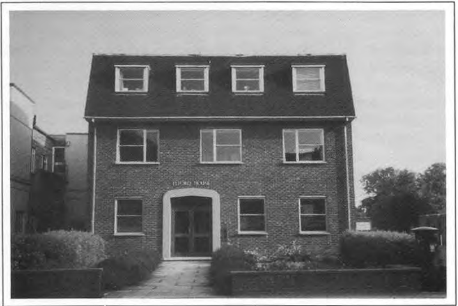
Elford House, 36 West Bar, Banbury, Aplins' office since 1972.
