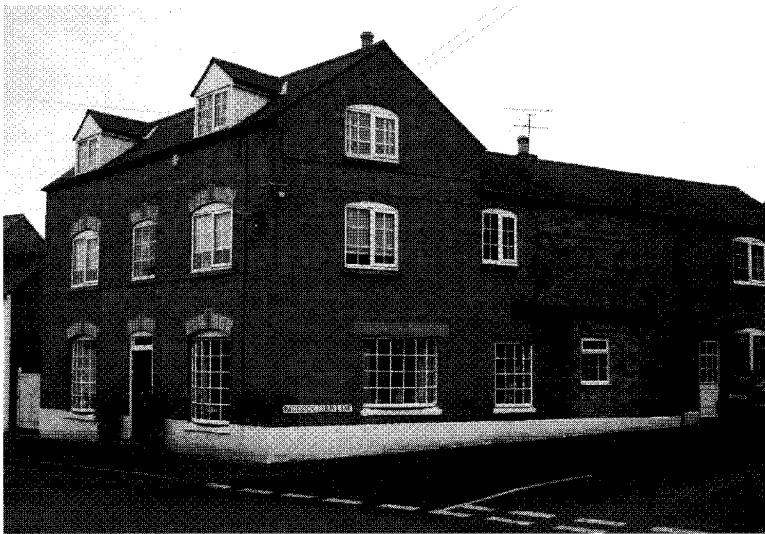
The building in its present state, with bowed windows and roof lights. The shop door is now a window; however, the brickwork at the side of the house reveals where the old wooden doors of the storeroom once were.
