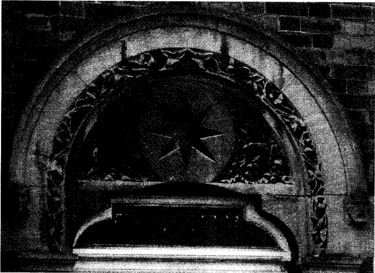
West Street, south end, Star Building House, built for Farmer Atkins.
