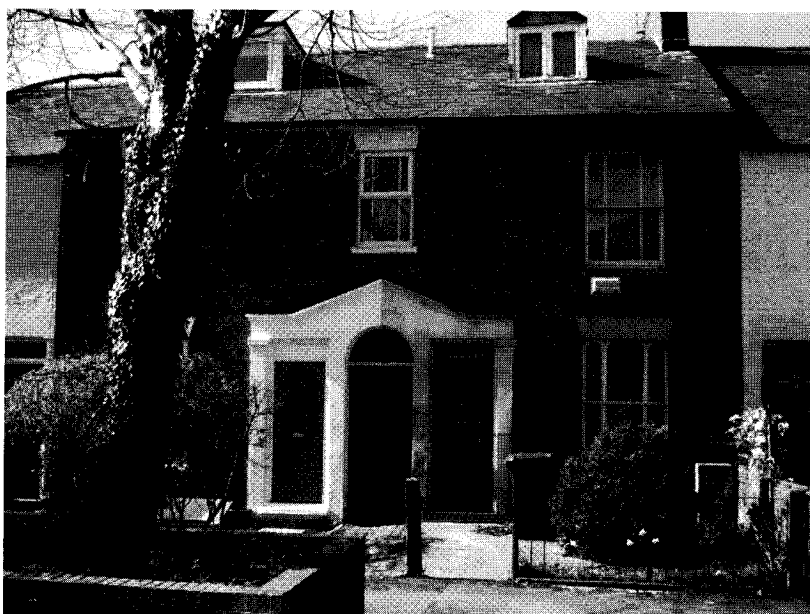
Original front door detailing, corner of Centre and South Streets.
