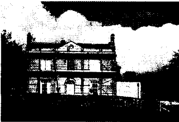
Fig 9. Holly House, Charlton, undergoing extensive refurbishment, 2009.
