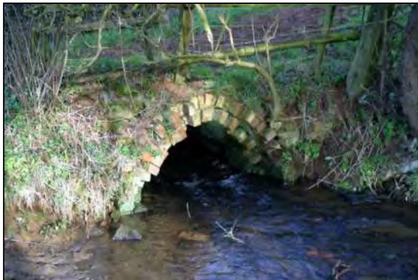
Footbridge over Sor Brook to Balscote.
