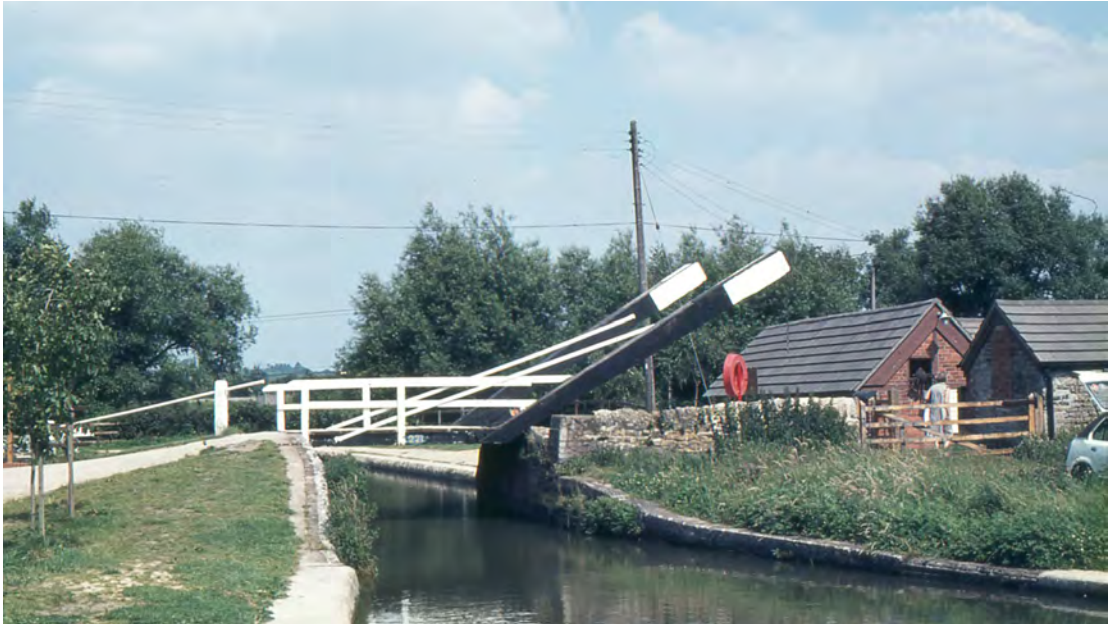
The Oxford Canal in the town and south of Banbury was characterised by lifting bridges, this example is at Thrupp
